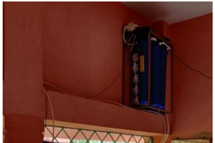
Heavy Duty Water filter, RCC Chandanpiri. 2019
