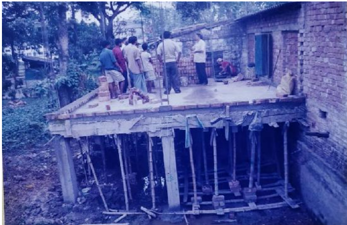
Construction work in progress, RCC Rasapunja. 2004
